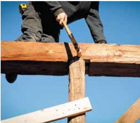
The barn's frame was made up of four large, H-shaped "bents" of columns, beams and Y-braces. A team of Mennonite craftsmen hoisted the barn at its new location, piece by piece as it was done a century and a half ago. All the structural elements in the house are original to the barn.
